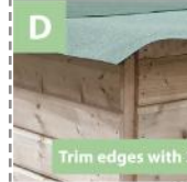
Neaten & cut excess felt
