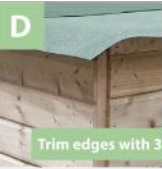
Neaten & cut excess felt
