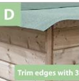
Neaten & cut excess felt
